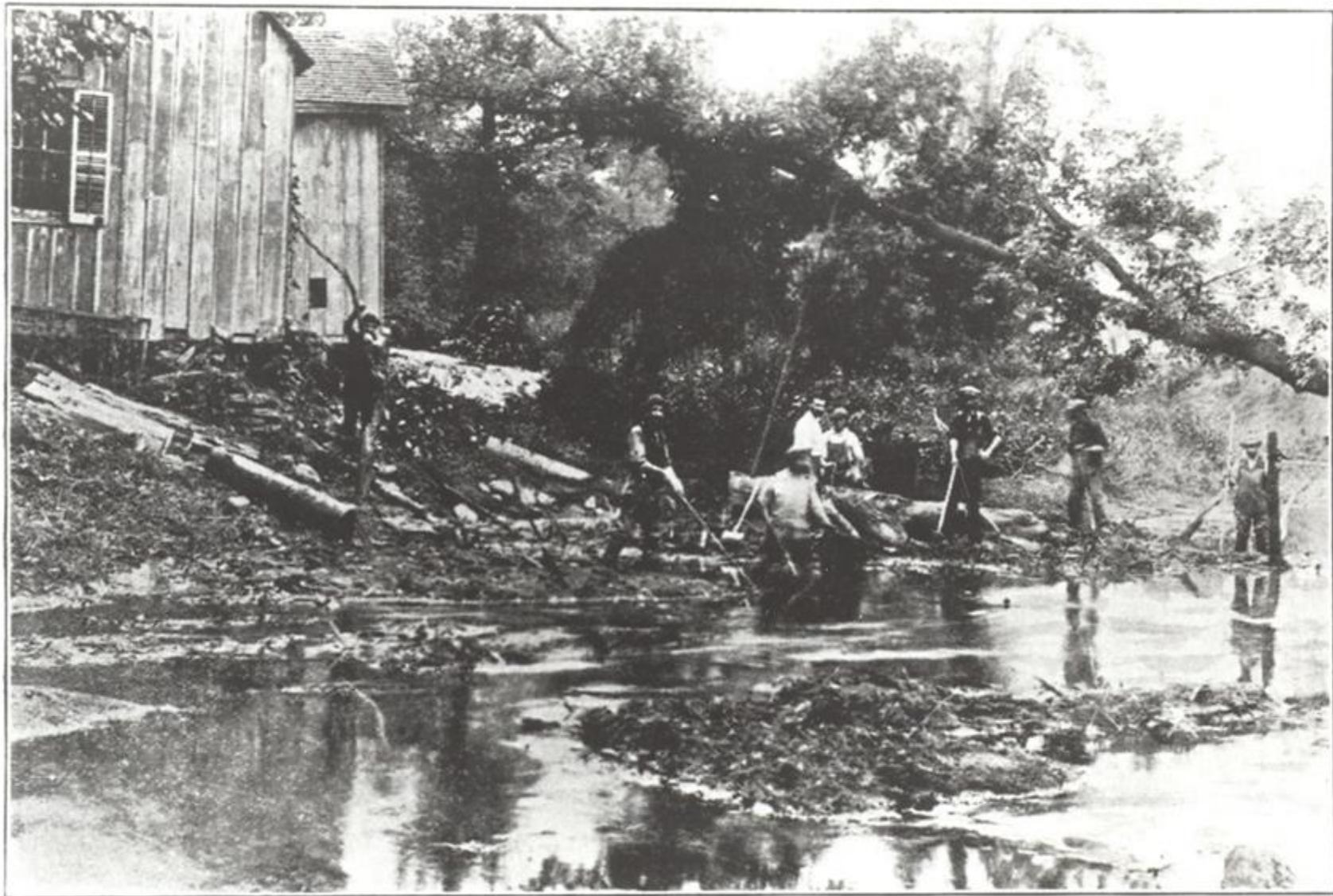
CLEANING THE RIVER PREPARATORY TO DEVELOPMENT SHOWN BELOW
